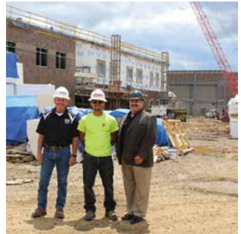
Grads at the building site: Project Manager - John (Shorty) May (1977), Job Foreman - Adam Douglas (2002), Owner - Fred Horner (1974)
